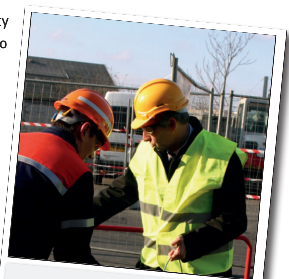
G. De Goyts, Works Manager, and J.P. Cleinec, President and General manager, laying the foundation stone
